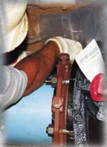
Uni-Flange Series 1500 Restrainer for PVC pipe.
