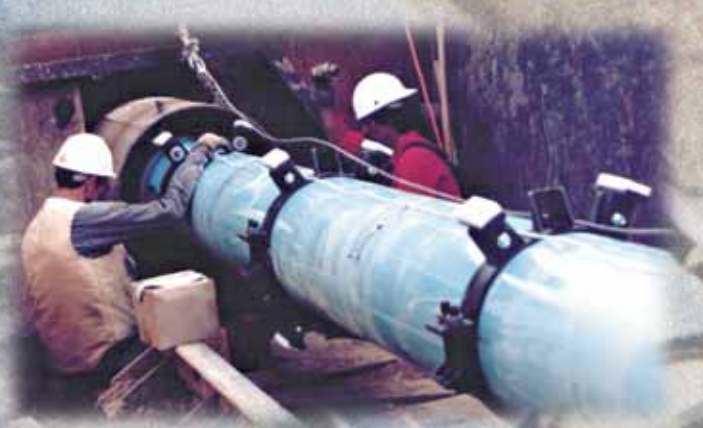
Uni-Flange Restrained Casing Spacers installed on 16" PVC pipe.
