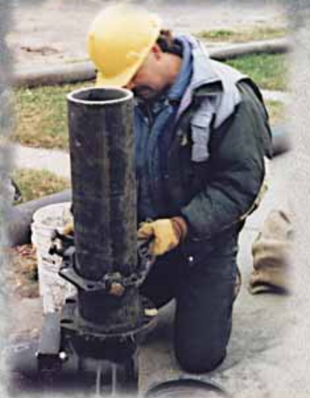
Uni-Flange Series 1400 Restrainer for ductile iron pipe.
