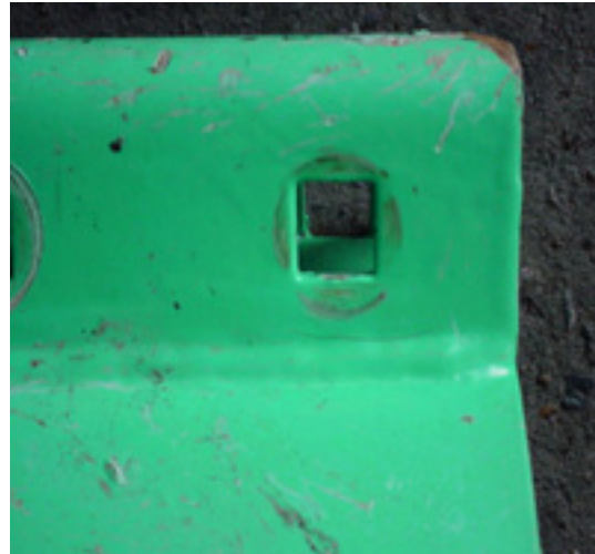
Epoxy coating damaged
